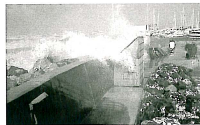
Fig. 5c Wave overtopping at Ostia (Italy).
